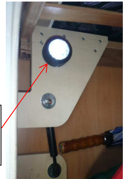
Added LED light in under-bed storage area
