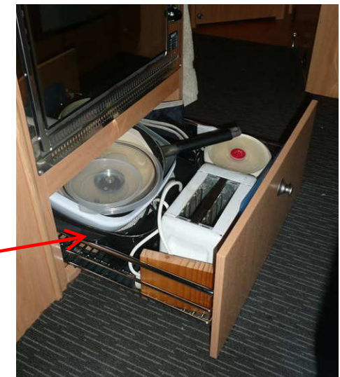
Converted cup- board under oven to a drawer [to im- prove accessibility; uses bottom runners]
