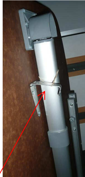
Added bracket under table to hook table to sliderail when not in use
